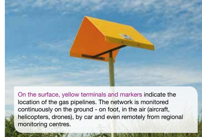
On the surface, yellow terminals and markers indicate the location of the gas pipelines. The network is monitored continuously on the ground - on foot, in the air (aircraft, helicopters, drones), by car and even remotely from regional monitoring centres.
