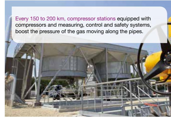
Every 150 to 200 km, compressor stations equipped with compressors and measuring, control and safety systems, boost the pressure of the gas moving along the pipes.
